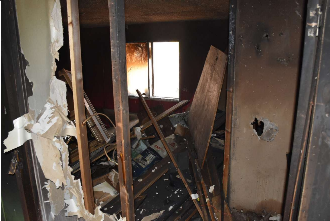
Figure 4 Photograph NJF_0020, West bedroom with storage
