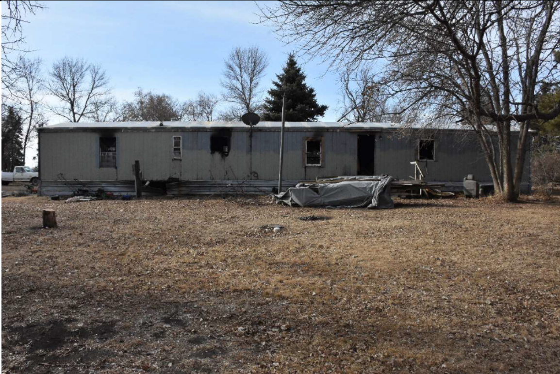
Figure 1 Photograph NJF_0001 North side of the structure
