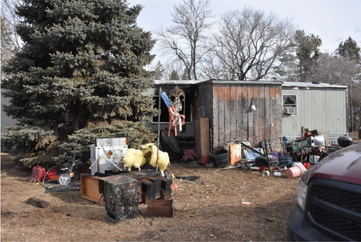
Figure 3 Photograph NJF_0011 South side of the structure
