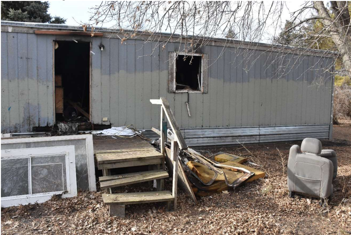
Figure 2 Photograph NJF_0005, North side of structure with door removed
