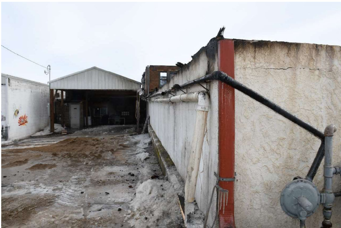
Figure 4 Photograph DSC_0034.JPG Exterior South Side
