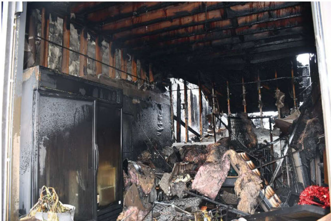
Figure 5 Photograph DSC_0061.JPG Interior Southeast Room
