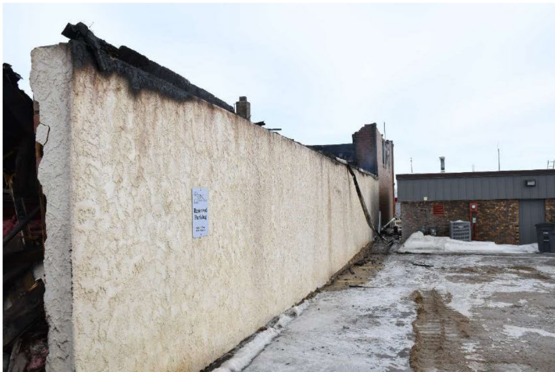
Figure 2 Photograph DSC_0008.JPG Exterior North Wall
