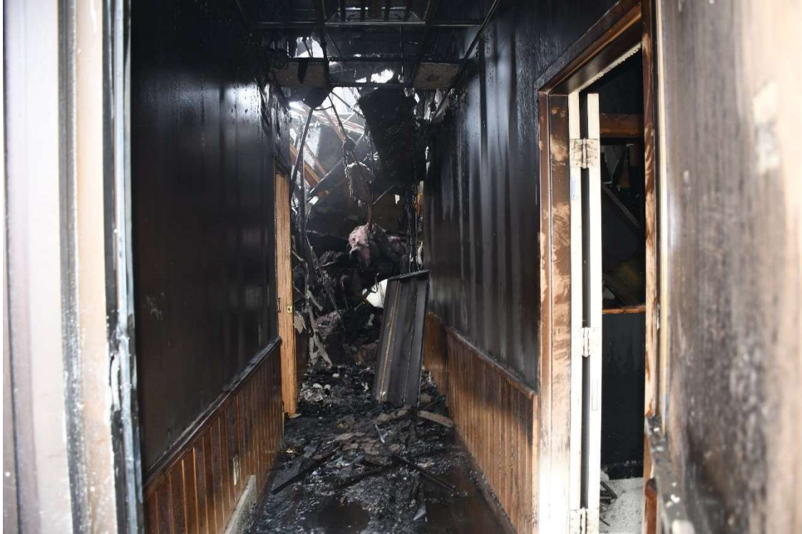
Figure 8 Photograph DSC_0084 Interior North Hallway
