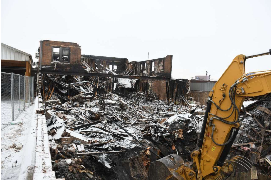
Figure 9 Photograph DSC_0008.JPG Exterior West Side
