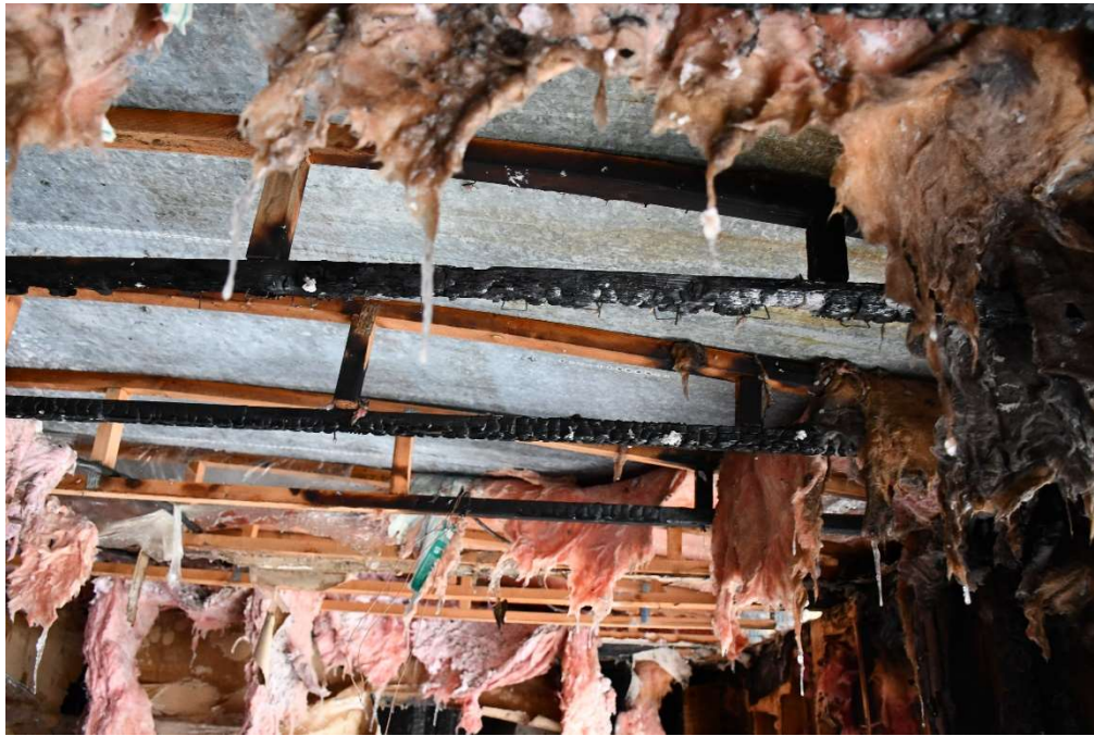
Figure 8 Photograph DSC_0091.JPG Truss Above South Bedroom Floor Door Opening
