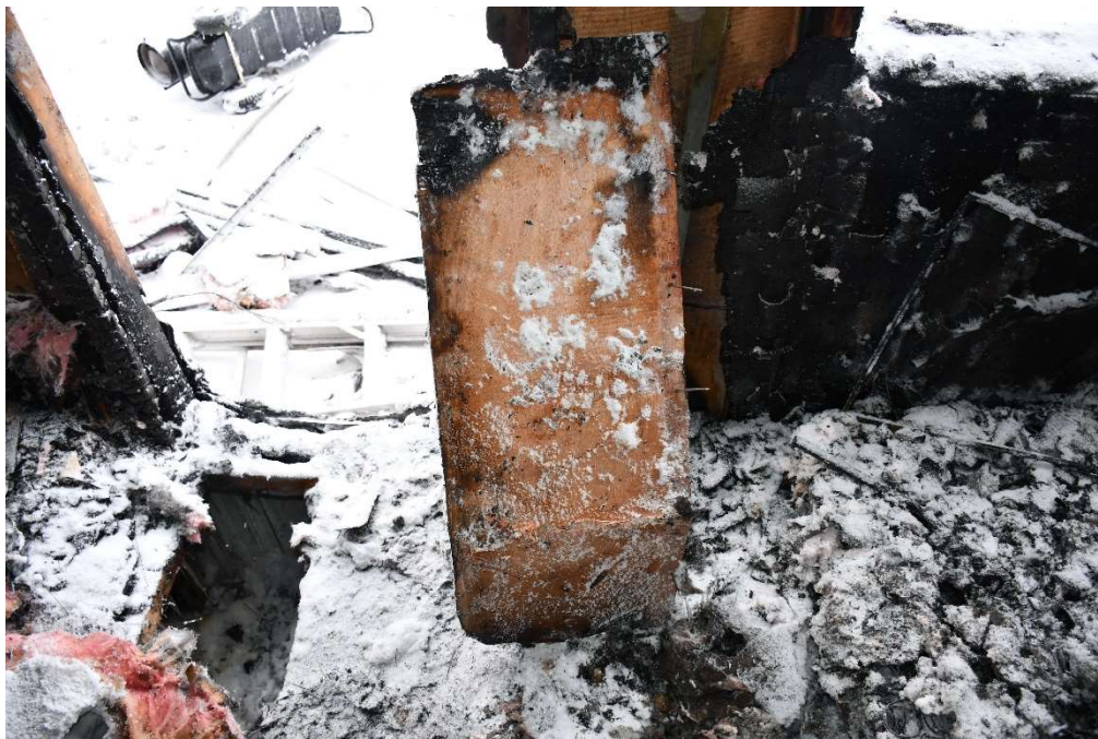
Figure 9 Photograph DSC_0098.JPG Bottom Side Of The Door For Floor Opening
